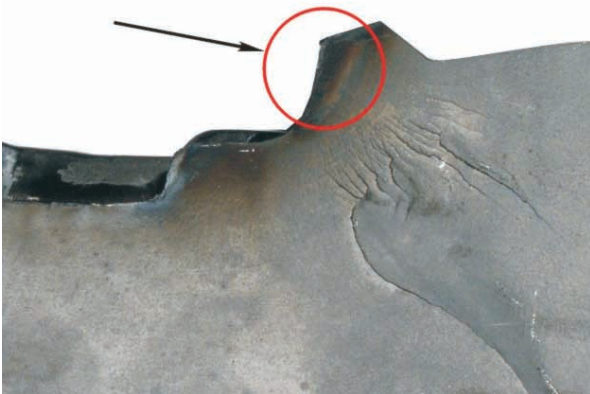
Fig. 2. Place of crack initiation
