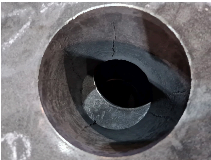
Fig. 4. Test casting B
